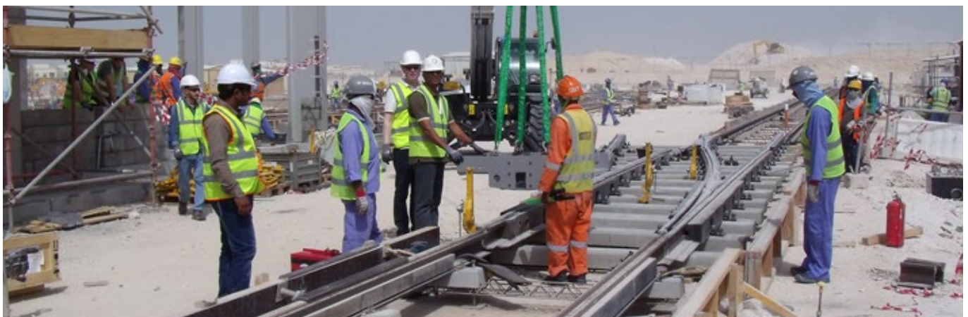
Assembly of point machine HW(E) 61.1 in the entrance to the depot
