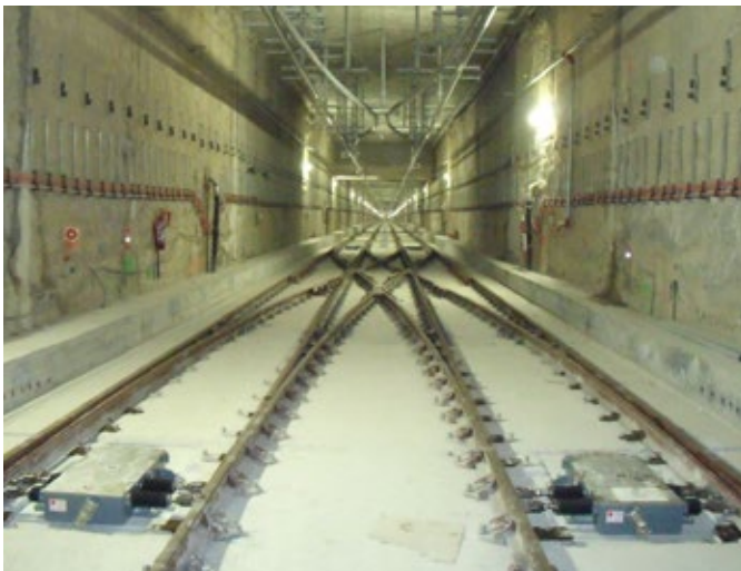
Point machine HW(E) 61.1 for a tunnel application
